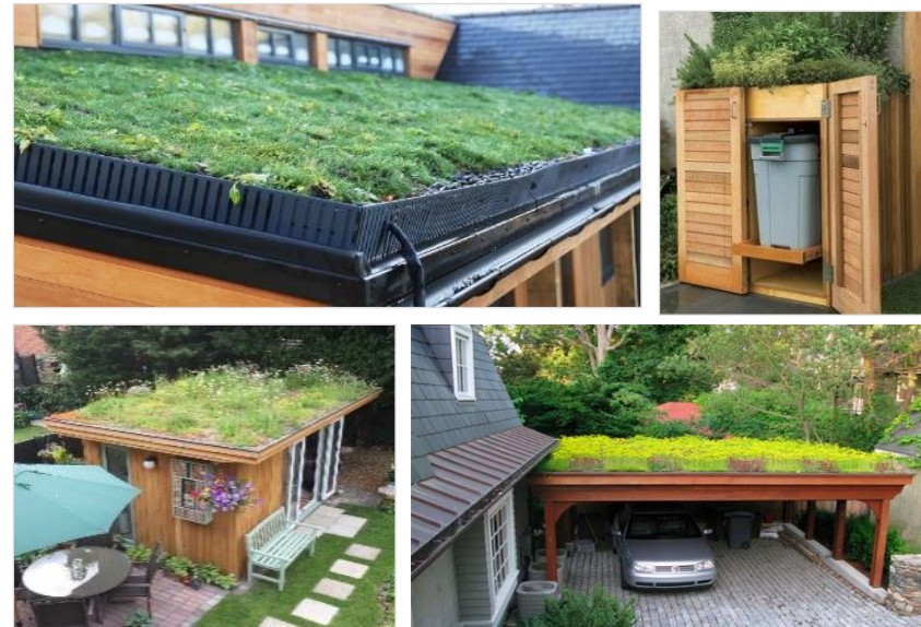
Green roofs can be applied to a number of flat or shallow pitched structures - extensions, sheds, stores and garages or car ports
