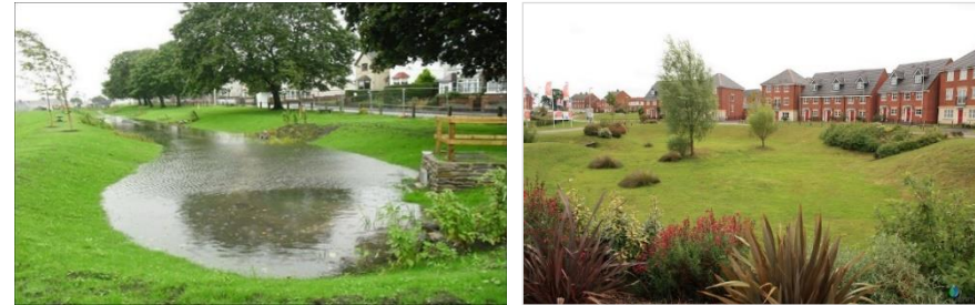
Filled detention basin served from swale and separate underground SuDS outlet pipe (left) and a dry detention basin with planting (right) adding to local character, biodiversity and providing amenity space
