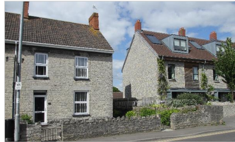
Infill development that provides a subtle updating of the local vernacular whilst following the established building line and scale.
