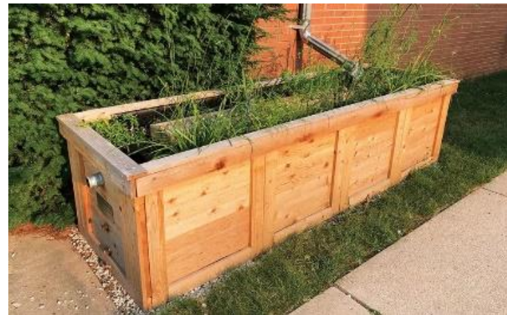
Rain gardens can be surface level and include water butts (top) or provided as planter boxes (bottom)
